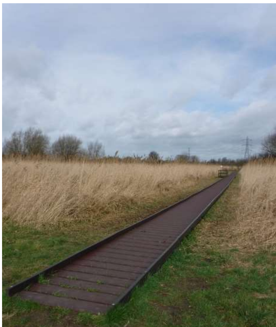
The New Boardwalk across the Reed Beds, Chertsey Meads, March 2017
